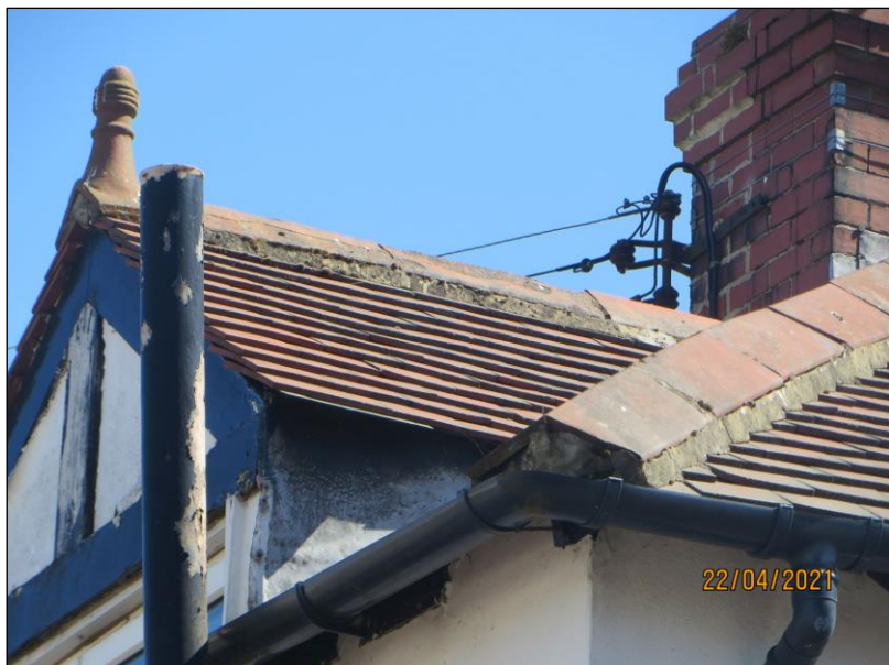
Figure 13. Close-up of roofline to the front of the property.
