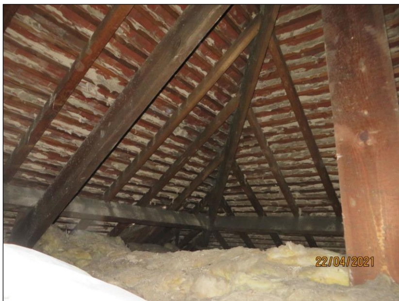
Figure 15. Loft void within property.
