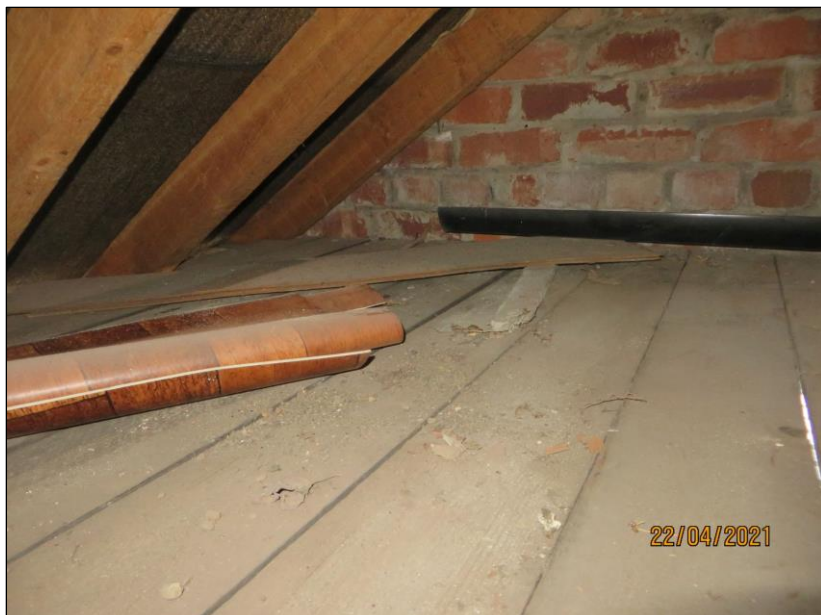
Figure 19. Storage area above garage space.
